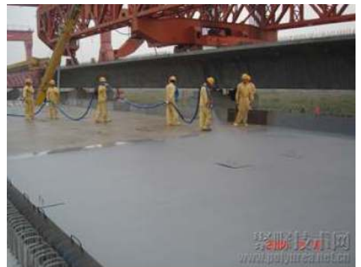
Lift the beams coated with polyurea on the pier
