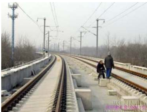
Lay the steel rail on the polyurea surface with 30mm asphalt emulsified asphalt sand
