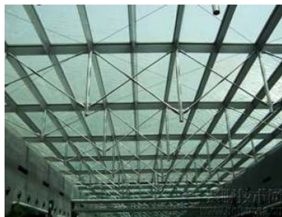
Water Pool Bottom with Black Polyurea
