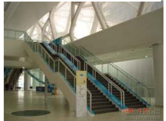
Floor and Stairs with Grey Polyurea
